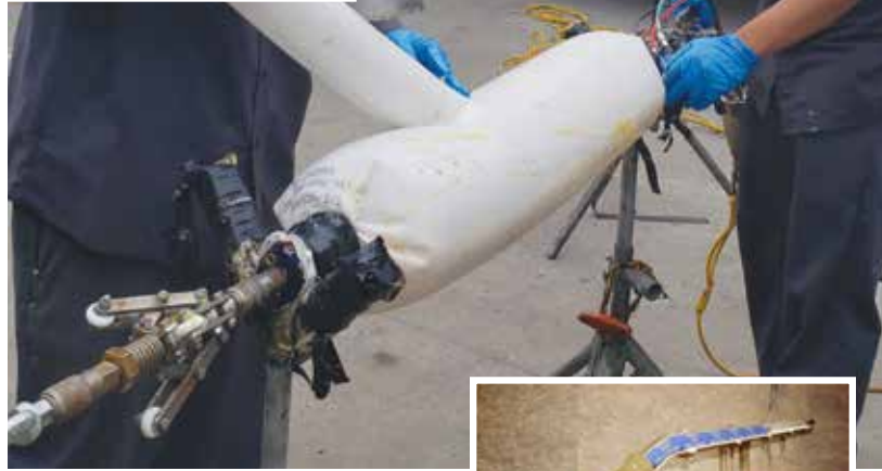
Lateral can be lined in one step with a remotely operated inflatable packer
